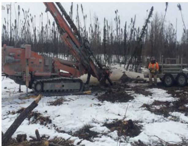
Photo 3: Directional drilling operations.
