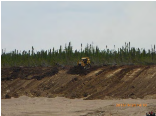
Photo 4: Spreading stockpiled soils over borrow pit slopes for rehabilitation.
