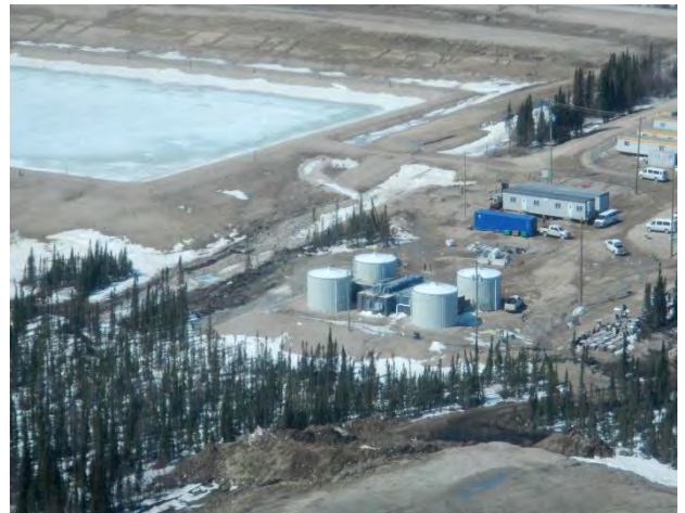
Photo 4: Hazardous material, septic and solid waste a safe distance from camp.
