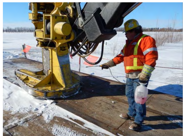
Photo 4: A worker disinfecting equipment to prevent the spread of bio-hazards.
