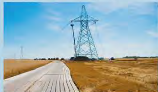
Bipole III transmission line construction
