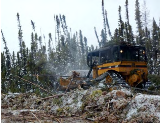
Photo 1: Clearing during frozen ground periods to minimize soil and vegetation disturbance.
