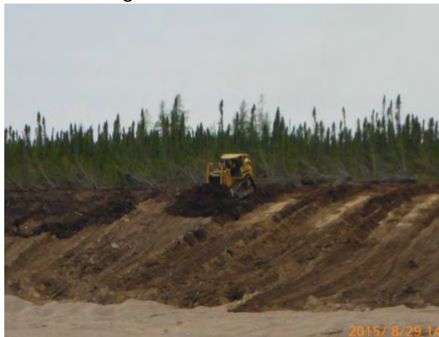
Photo 3: Stockpiled soils are placed over the edges of a borrow pit.
