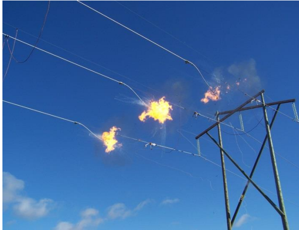
Photo 1: Conductor splicing using implosion sleeves.
