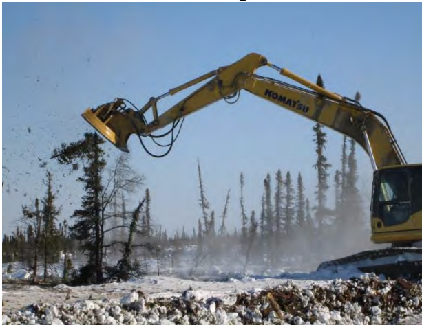
Photo 3: A danger tree is carefully removed to prevent impacts to soils and adjacent vegetation.
