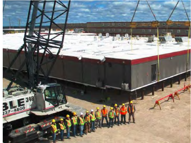
Photo 2: Construction of the Keyask workcamp.
