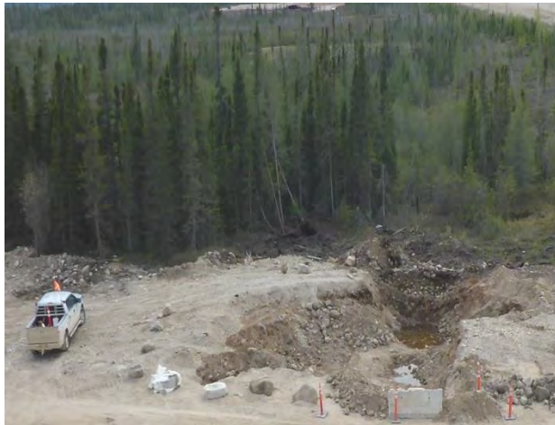
Photo 1: The excavation of a petroleum fuel storage area at Keewatinohk.
