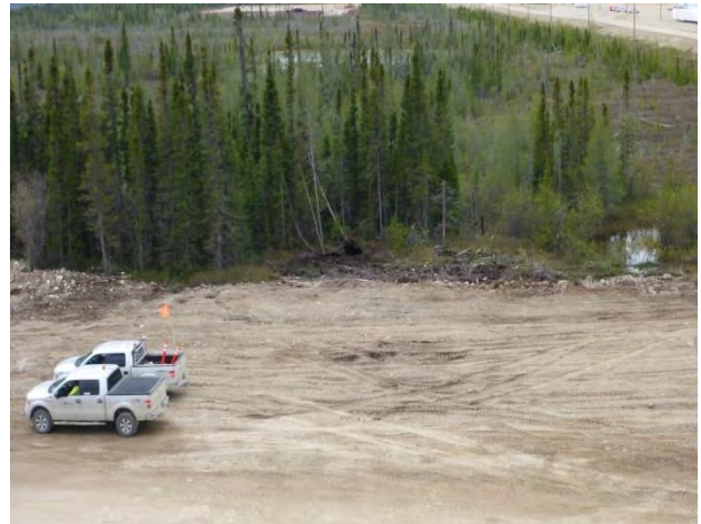
Photo 2: After the excavation of a petroleum fuel storage area at Keewatinohk.
