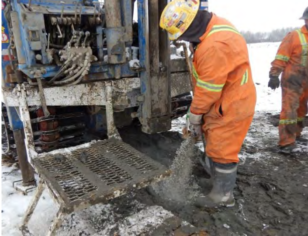
Photo 5: A drill hole being sealed with bentonite to prevent water contamination
