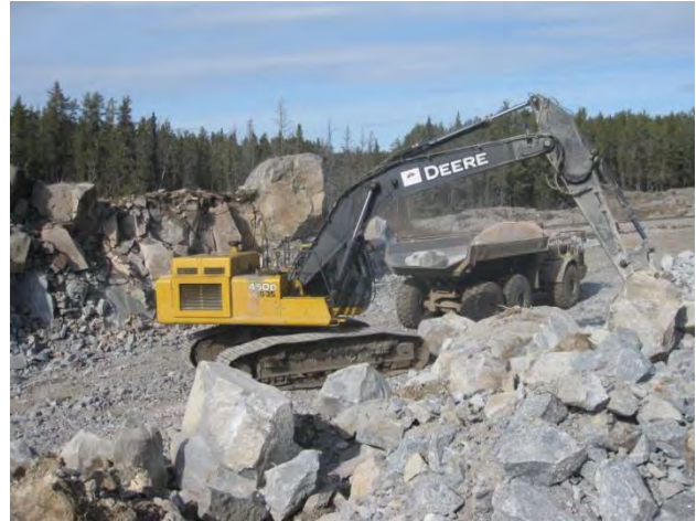
Photo 2: Rock is blasted and quarried for project use.
