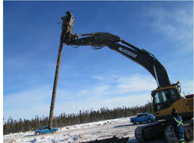
Photo 2: Drilling equipment being inspected regularly for fuel and oil leaks and spills.
