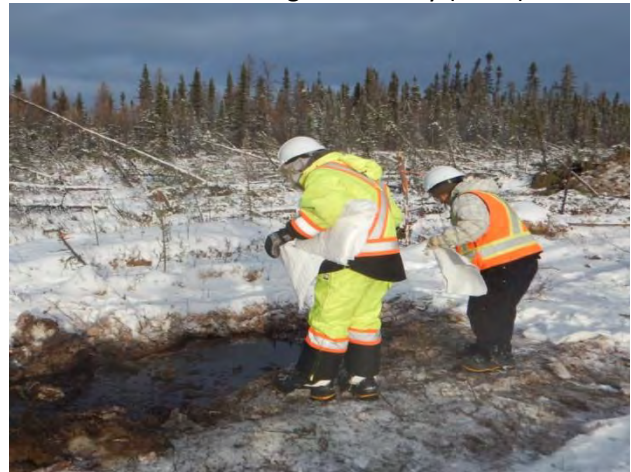
Photo 4: A fluid leak from a piece of machinery is contained.
