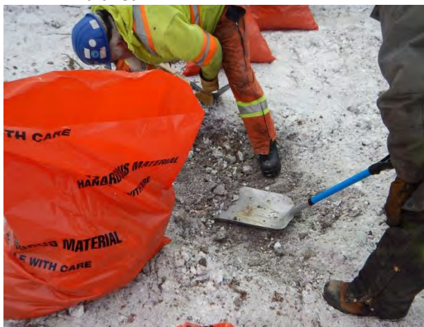
Photo 5: Contaminated soil is removed by shovel.
