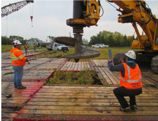
Photo 1: Low disturbance methods for drilling.
