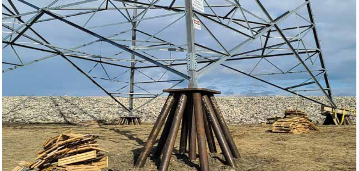
Debris near MMTP Tower 120 to be picked up for recycling/disposal. All debris is placed on a deficiencies list for clean up by contractors and checked by Manitoba Hydro or Compliance and Environment Monitors. This debris has now been removed from the ROW.
