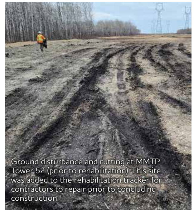
Equipment tire tracks within the "No Machine Zone" near water's edge on MMTP
